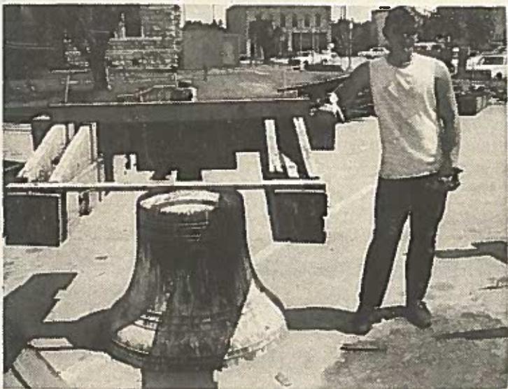
HOLLY WARREN OF WEATHERFORD STANDS BESIDE THE HUGE BELL HE AND OTHERS TOOK DOWN FROM THE GRANBURY COURT HOUSE. TIMBER SUPPORTS ON THE BELL WERE SECURED TOGETHER BY HUGE HAND-FORGED SQUARE NAILS.
